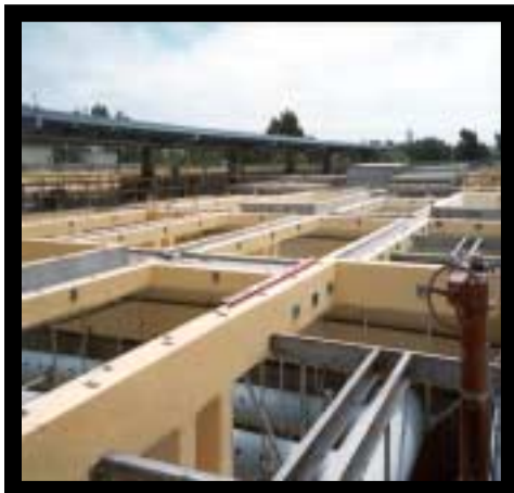
View of sedimentation basin coated with ECOSYSTEM® expanded EF-1988
