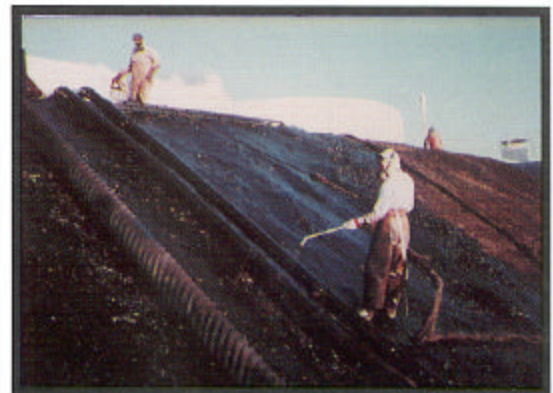
ECOSYSTEM ® expanded materials applied direct-to-earth for embankment stabilization. Minimal surface preparation required.
