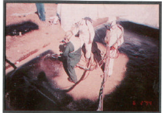
ECOSYSTEM ® process applied direct-to-earth for secondary containment liner.
